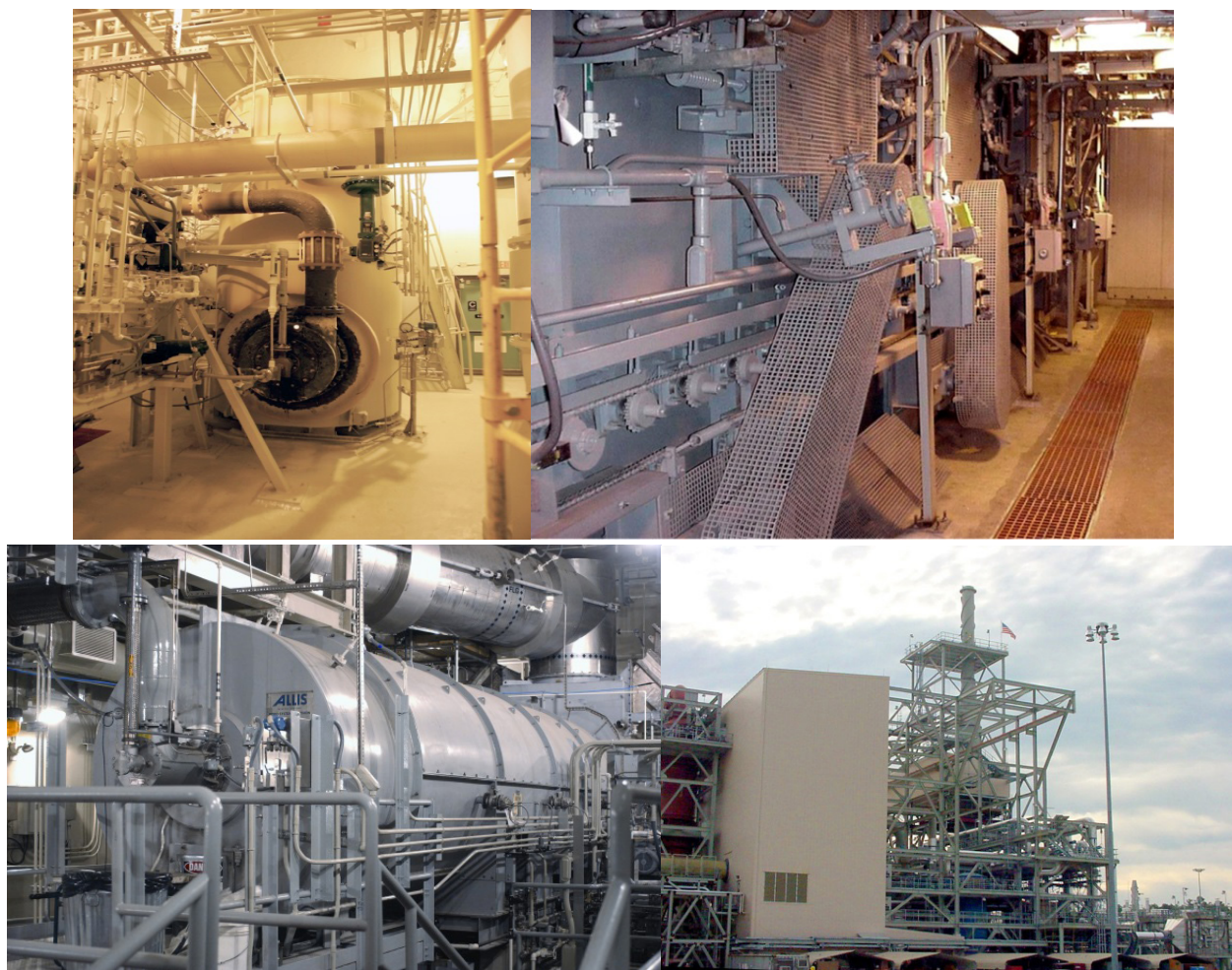
Figure 9.B. Facilities for chemical agent incineration operations. Top left: Liquid incinerator; Top right: Metal parts furnace; Bottom left: Deactivation furnace; Bottom right: Pollution abatement system.
